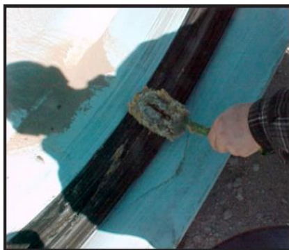
Lubricate gasket.
